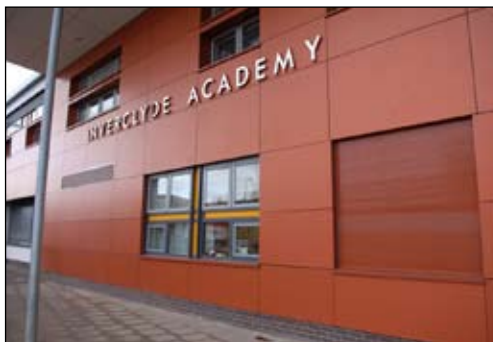
West Inverclyde Academy, Greenock, Scotland (2008): The extensive support offered to clients at every stage of the design and installation process was one of the reasons why Charter was awarded this prestigious contract.
